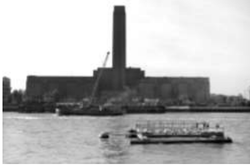
Şekil 15 – Bankside Power Station
